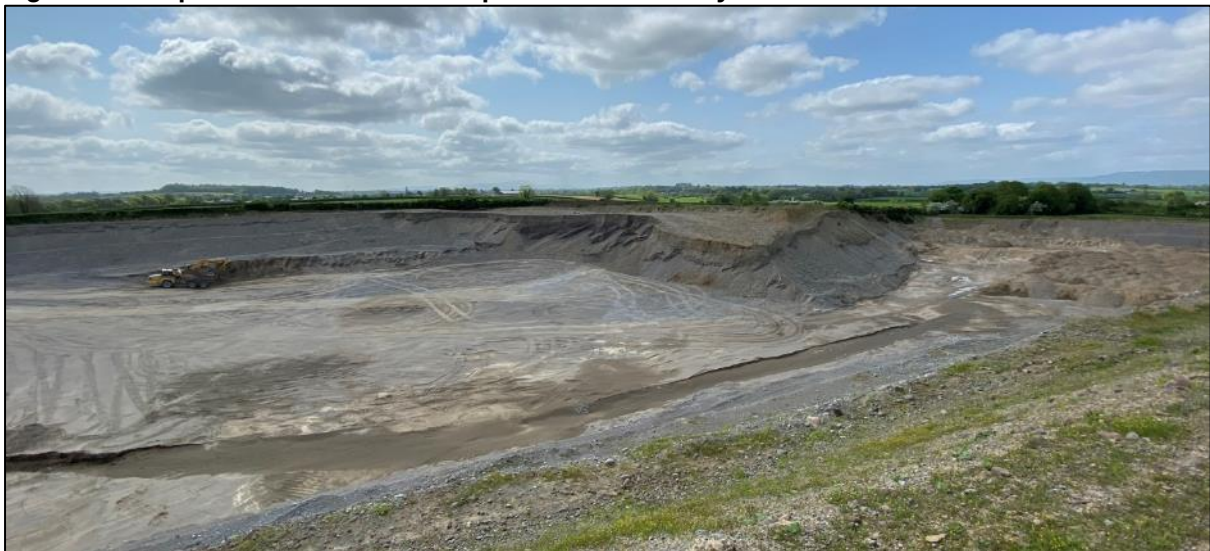
Figure 7-2: Exposed Sand and Gravel pit face within Ballyburn Pit
