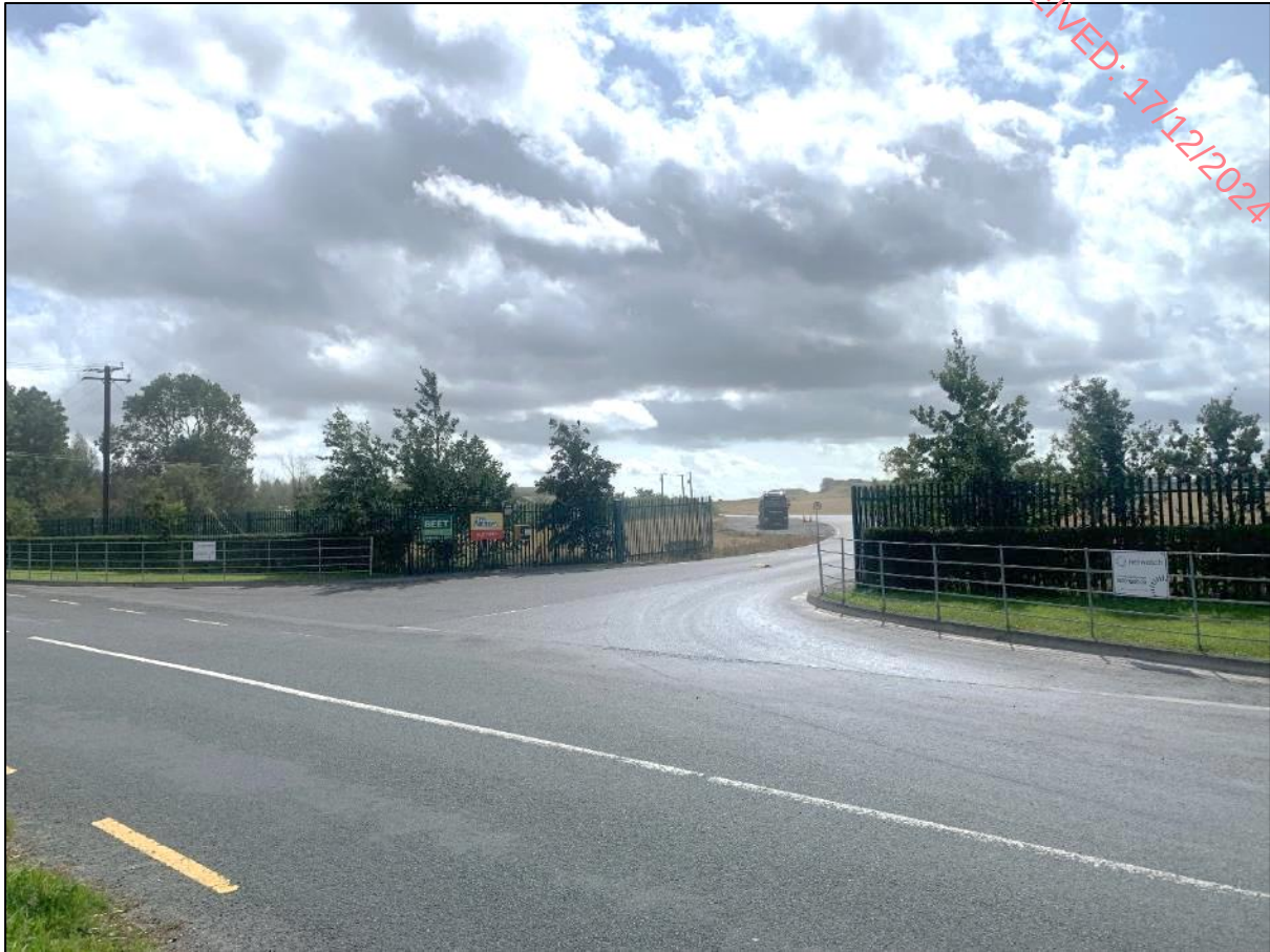
Plate 3-1: Site Entrance Gates
