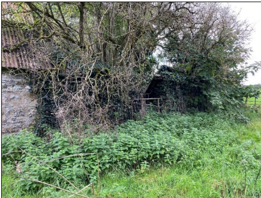
Plate 12-1: Structure 1 looking southwest
