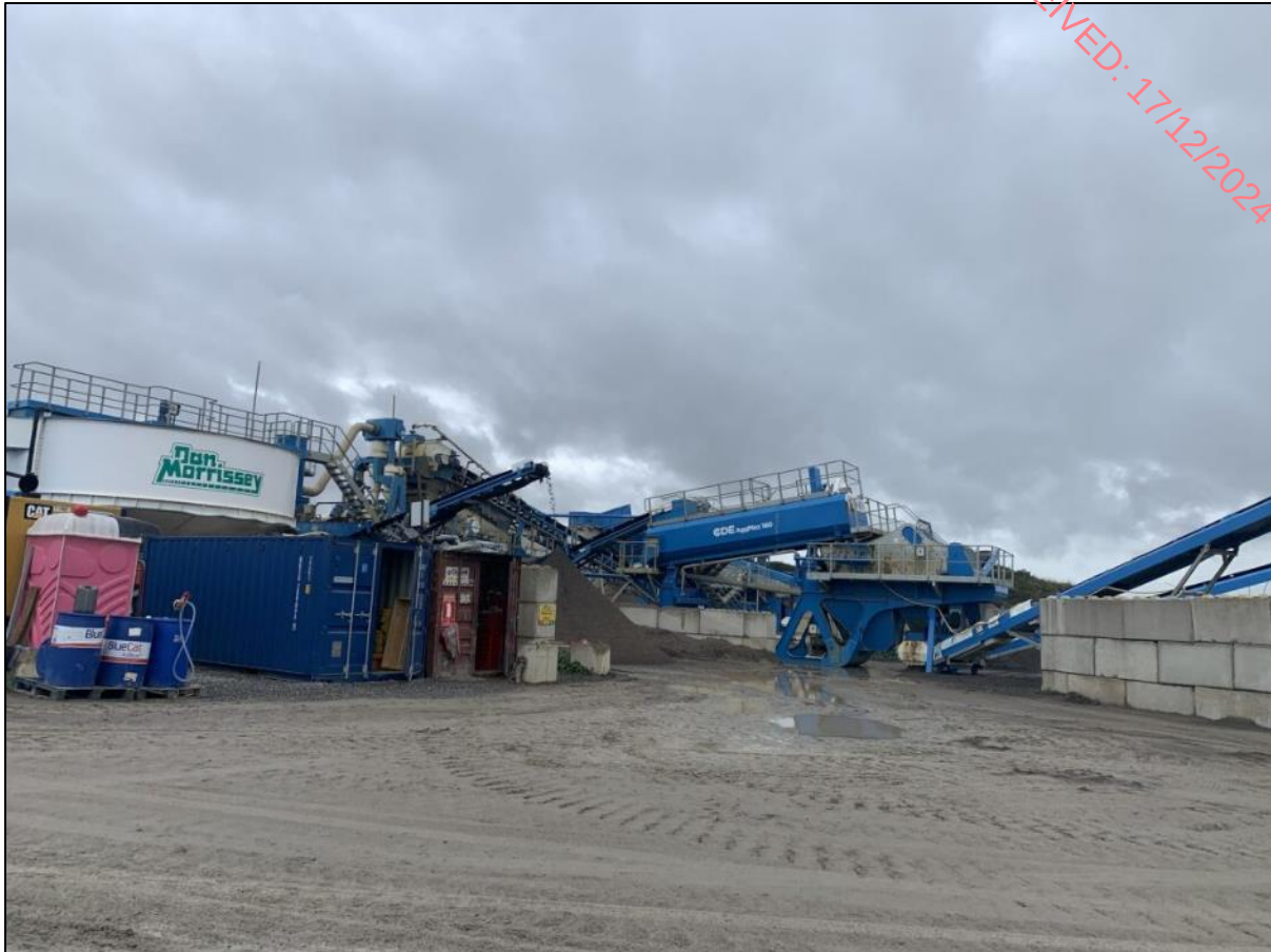
Plate 3-5: Existing Closed System Screening Plant with Workshop and Storage Bay
