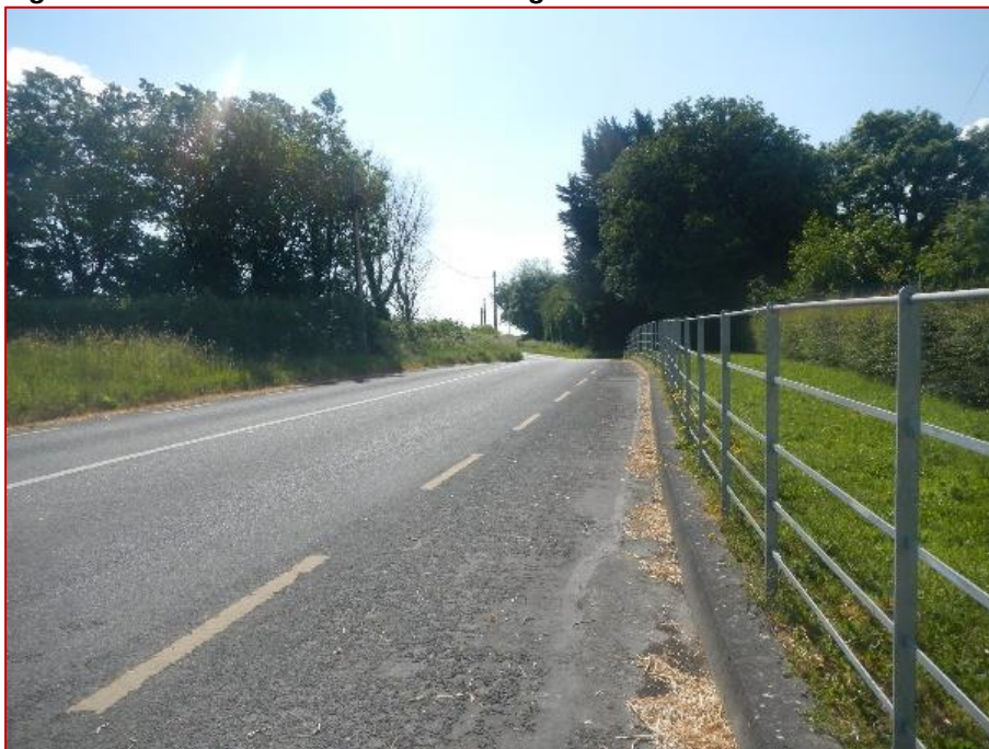
Figure 13-1: L4012 Local Road Looking Northwards
