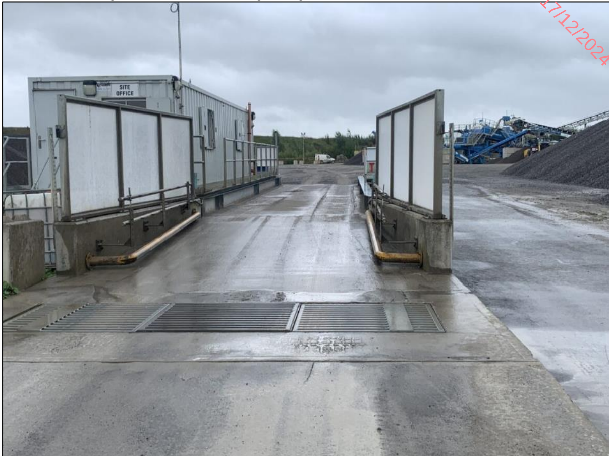
Plate 3-3: Existing Wheel Wash and Weighbridge
